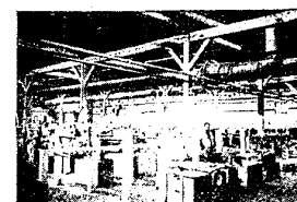
Ventilation, Humidification, Chauffage.
